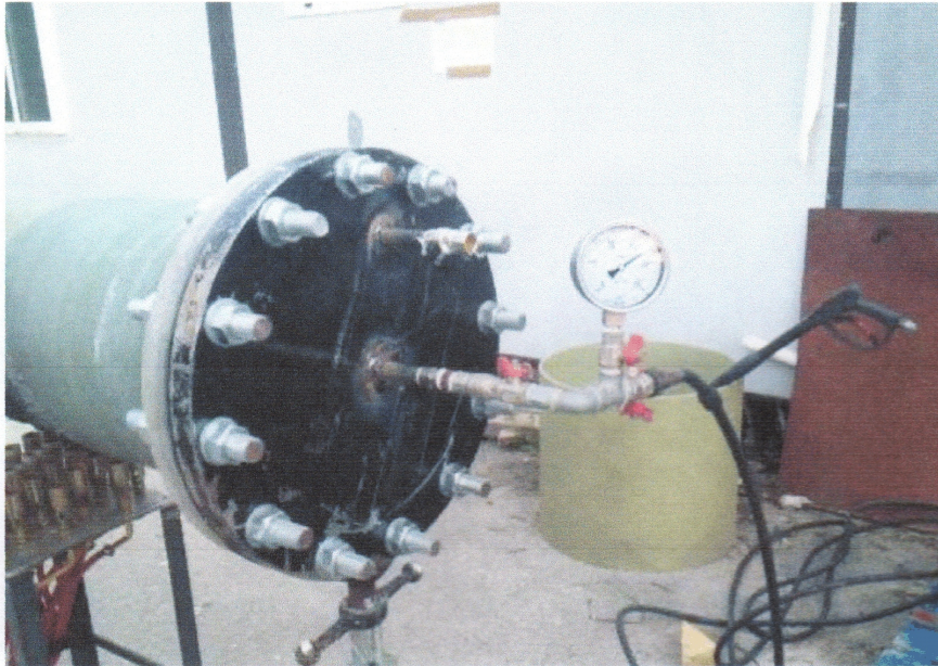
Picture no. 11: start of pressure test at 18 barg
